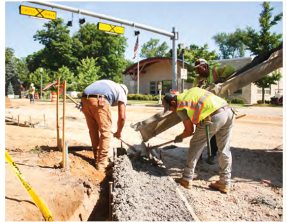
New concrete being poured for the curb and gutter
