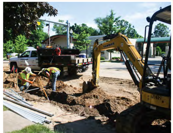
Construction underway opposite the Sam Corey Senior Center
